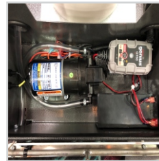
Battery Powered Pump Moves Finishes from Pail to Floor
